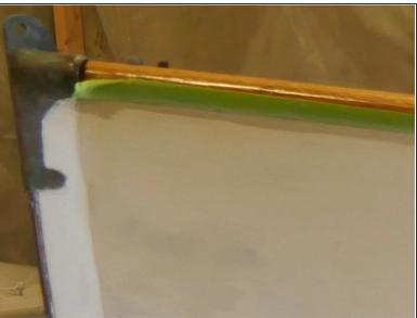
Apply a quick-release <u>masking tape</u> to protect adjacent surfaces.
